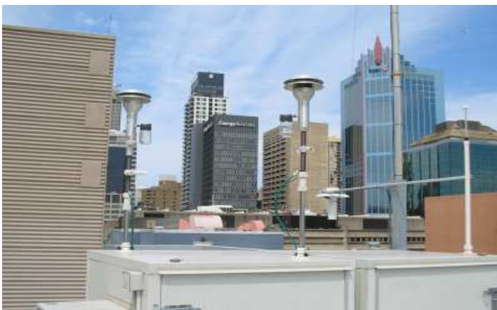
Ambient Air Quality Monitoring Station with the Sydney skyline in the background
