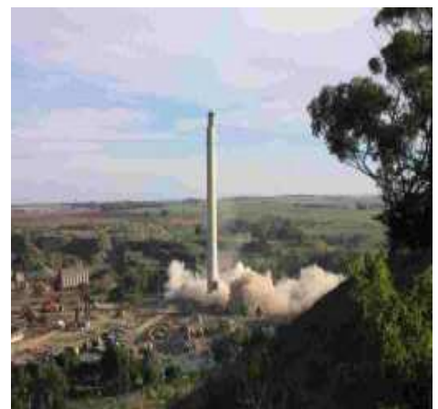
Destruction of Geelong Cement Stacks
