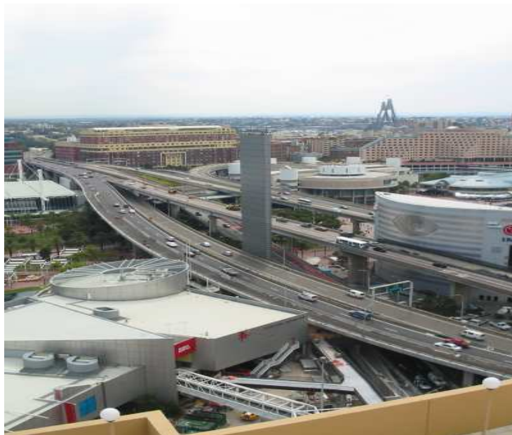
Cross City Tunnel Ventilation Stack
