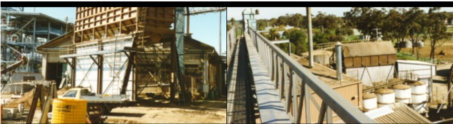
LEFT Meal storage and dust control systems under construction, Numurkah
